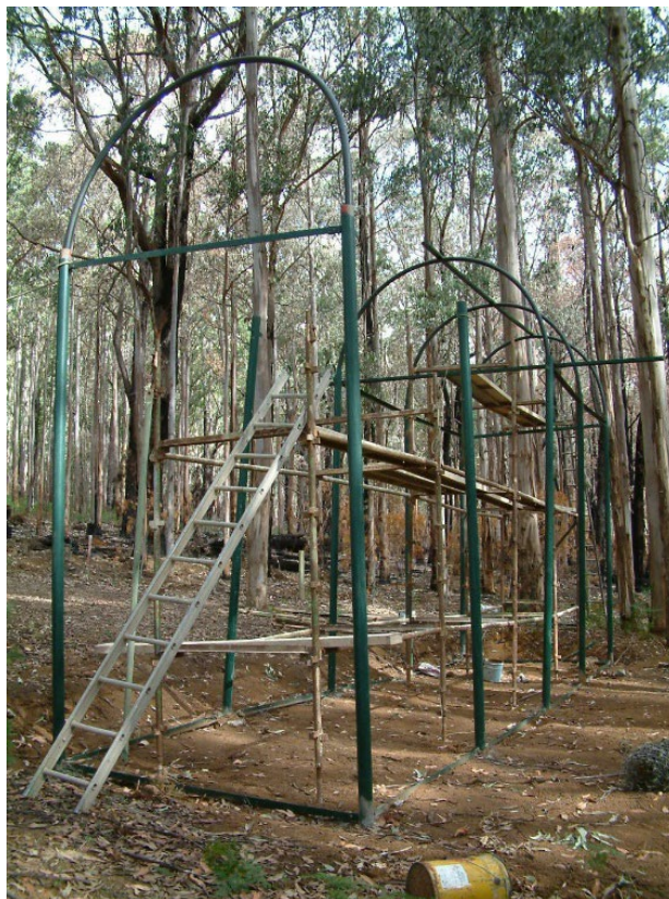
Figure 9.16 A pre-release aviary for gliders is shown under construction. Note the height required to permit gliders to be able to glide. Thin bird wire and shade-cloth are then used to cover the aviary.
