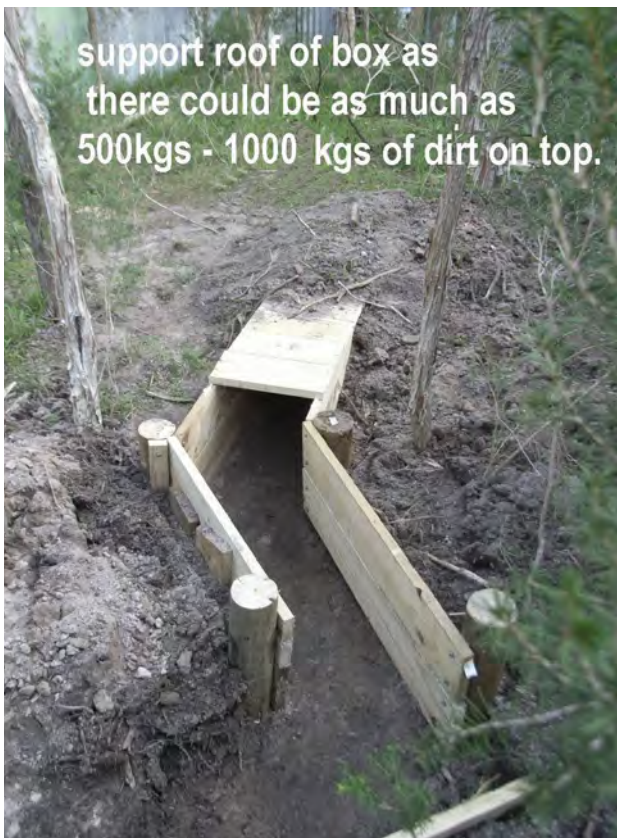
Figure 10.13 Artificial burrow entrances may need to be reinforced with wooden sleepers.
