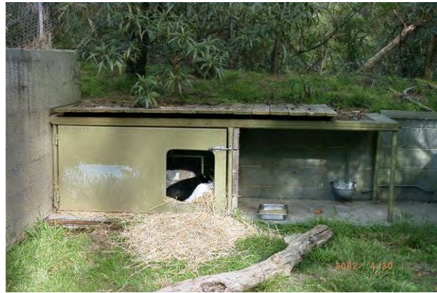
Figure 10.14 Pre-release wombat enclosure. Note solid walls, artificial den with door for easy access and food placed in a tray on concrete flooring for ease of cleaning and to minimise faecal build up.
