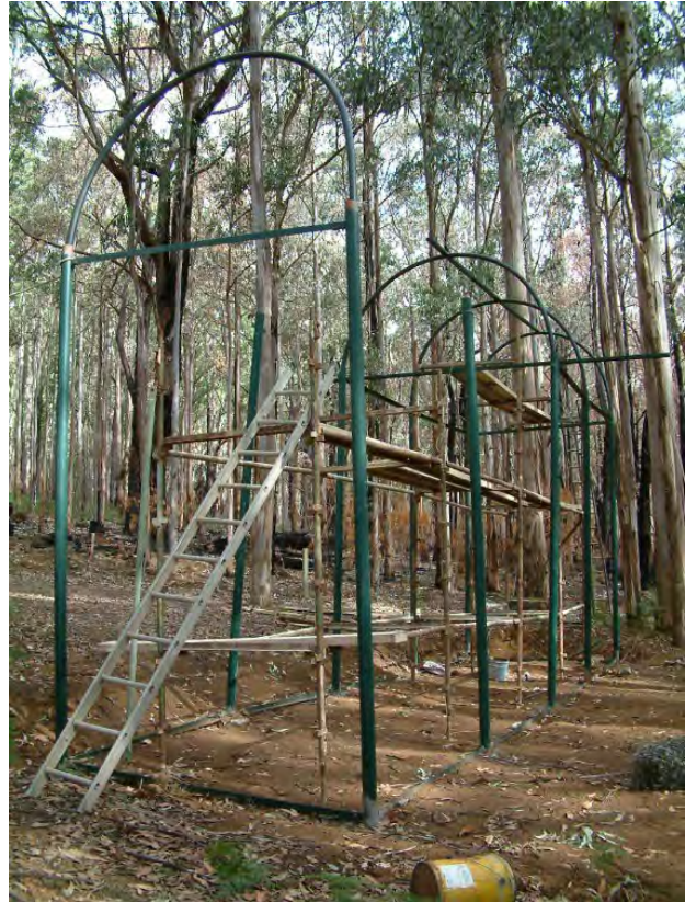
Figure 9.16 A pre-release aviary for gliders is shown under construction. Note the height required to permit gliders to be able to glide. Thin bird wire and shade-cloth are then used to cover the aviary.
