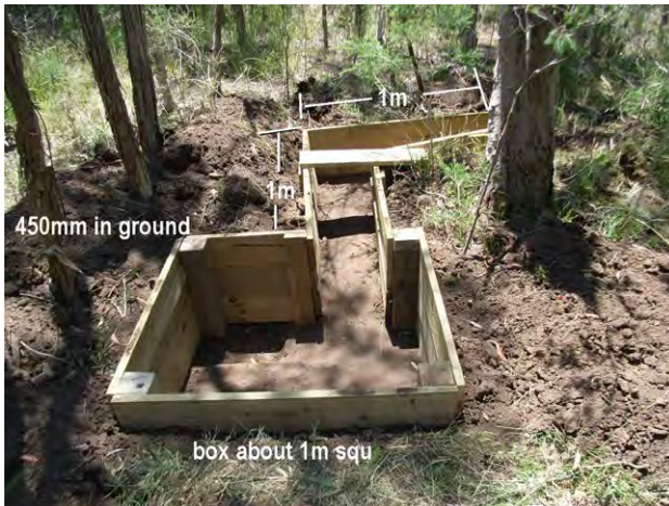
Figure 10.12 An artificial burrow under construction in a pre-release yard.
