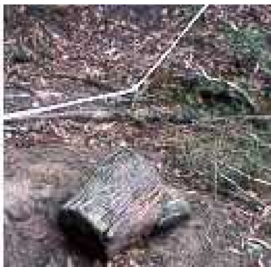
A log section has been used to anchor a corner in a single- strand electric fence.
